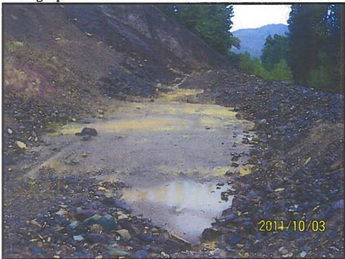
Photos of the constructed berm to comply with the perimeter fence requirement of the reclamation plan. Berm also serves as a storm water retention basin and provides for an added measure of safety to rock fall or slope failure.
