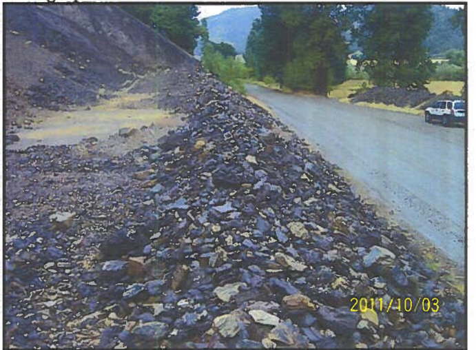
Photos of the constructed berm to comply with the perimeter fence requirement of the reclamation plan. Berm also serves as a storm water retention basin and provides for an added measure of safety to rock fall or slope failure.
